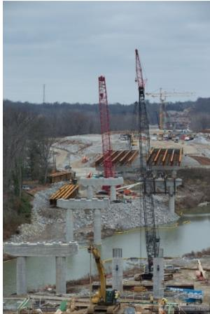
One of four bridges (Wolfpen Bridge) is complete on section 4 (Kentucky Side of River from I-71 to Ohio River) and work on Harrods Creek Bridge continues. Soil nail and rock anchor walls, concrete paving, Harrods Creek Bridge, and excavation and blasting are expected to continue throughout the summer.
